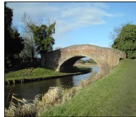
Colton Turn-over Bridge.
