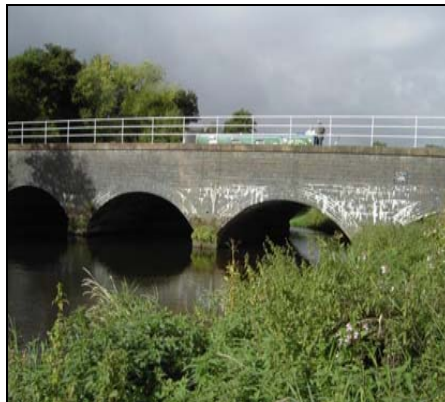
Canal aqueduct over the River Trent.
