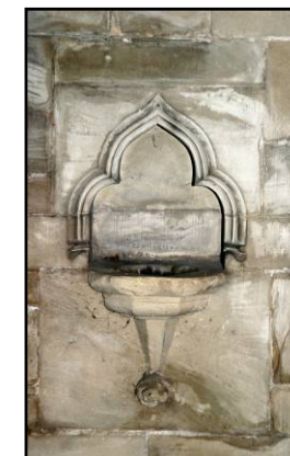
The piscina found in the present chancel.
